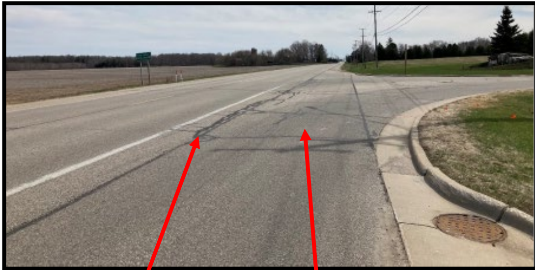
Transverse Cracking
